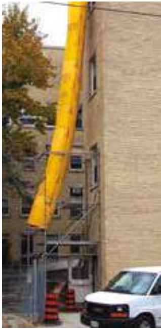
TYPICAL INSTALLATION ON SYSTEM SCAFFOLD
